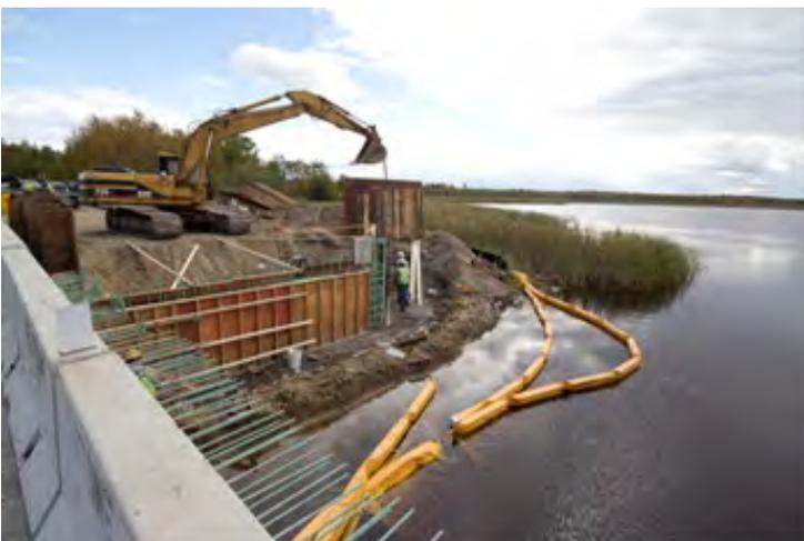
**Use floating silt curtain for work in the water as secondary containment to contain sediment close to the work area.**
