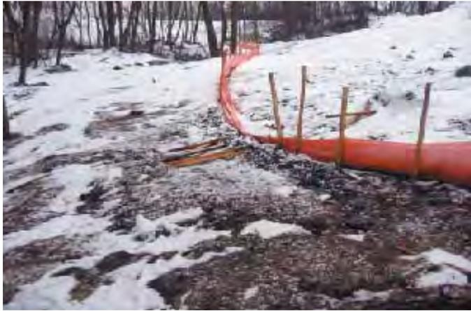
If construction is going to continue during the winter and new areas will be disturbed that requires new sediment controls; materials such as compost berms, logs and rolls, fiber rolls, rock bags and rock filters can be installed over the snow cover. These installations will need extra care and frequent inspections to assure continued effectiveness.
