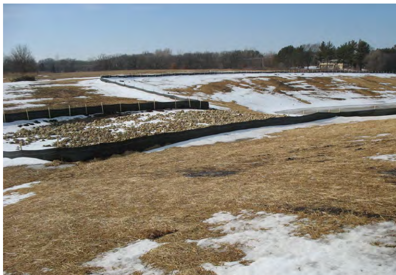
Silt fence used as perimeter control
