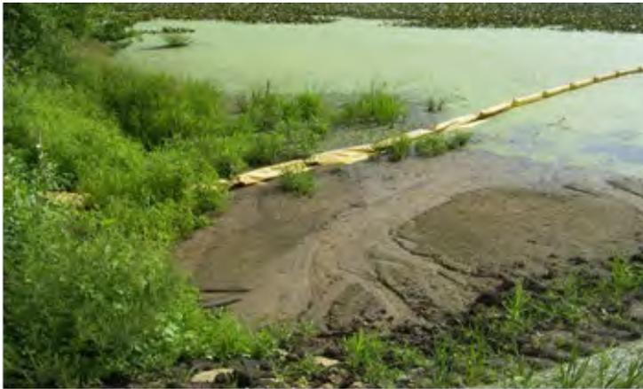
**Relying on floating curtain as down gradient perimeter control will result in permit violations for failure to install sediment control and in most cases will result in water quality violations.**
