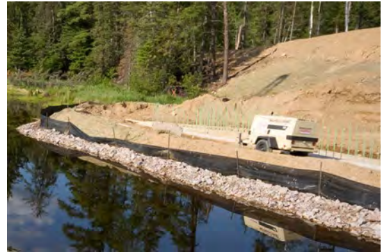
Move perimeter controls up the bank as the bank is stabilized.
